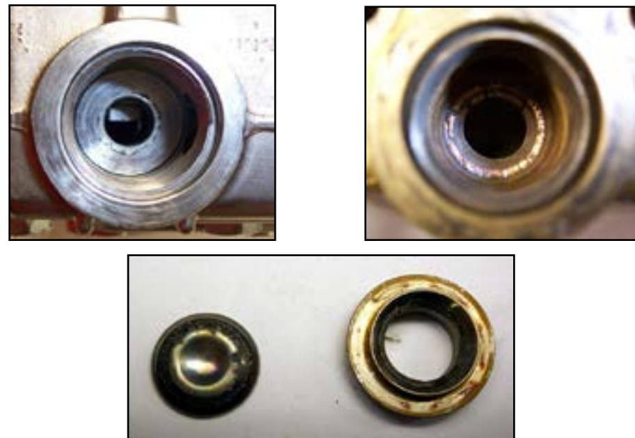
Figure 5-2. Inspect Manifold and Old Valves
